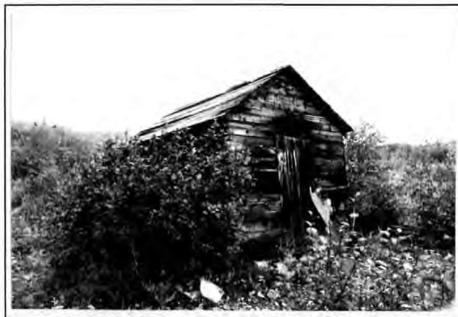
Figure 156. The Parts Shed, 1993. The view is looking northeast.
